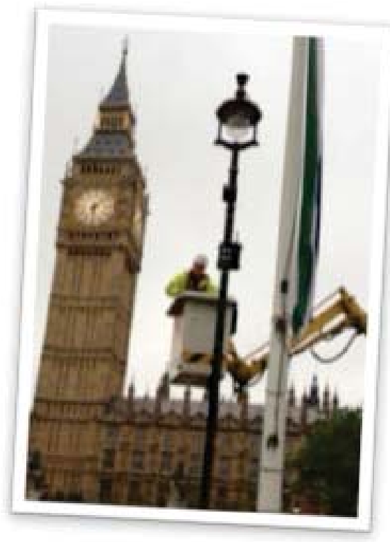
Figure 8 Light pole mounting a Wi-Fi AP and a small cell
