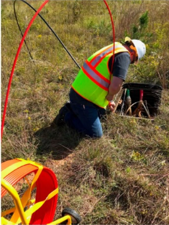
Rodding thru the Coax + Conduit
