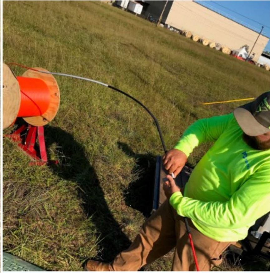
Attach the micro duct
