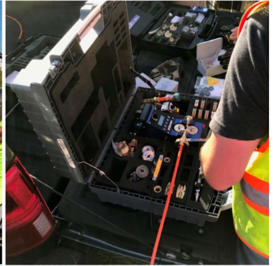
Push Fiber thru the 806 ft Plumettaz/U E101
