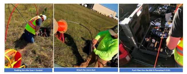
Figure 7 – Illustraing the Rod-and-Rope process and blowing fiber into the installed micro-duct
