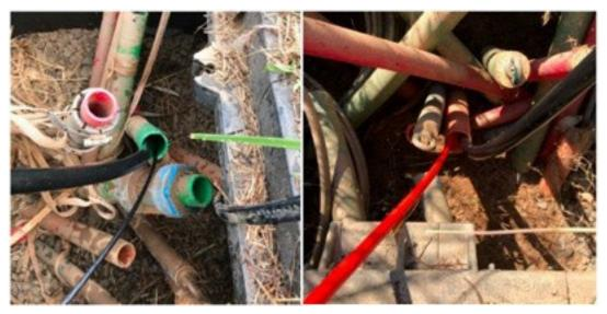
Figure 8 – Finished micro-fiber and micro-duct installed
