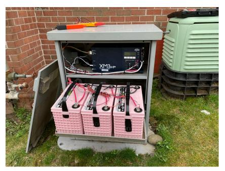
Figure 3 – Pad mounted Outside Plant with Batteries Shown
