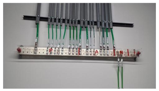
Figure 3 – Master Ground Bar With PANI Configuration
