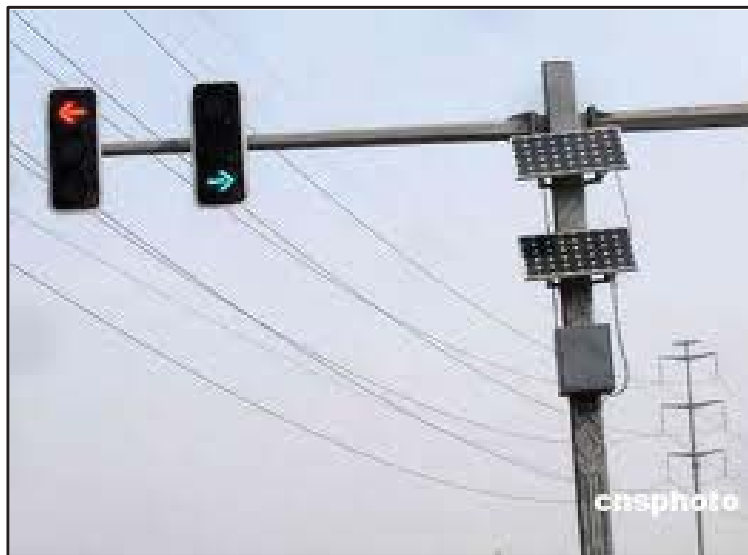
Figure 10 – How Far Can Cable Take “Green” in the Outside Plant?
