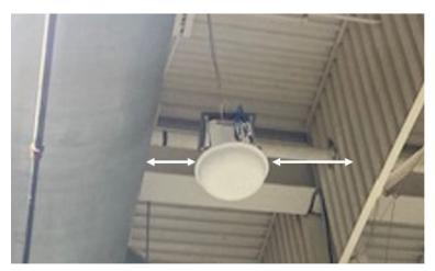
Figure 10 - Antenna blocked by metal duct and rail
