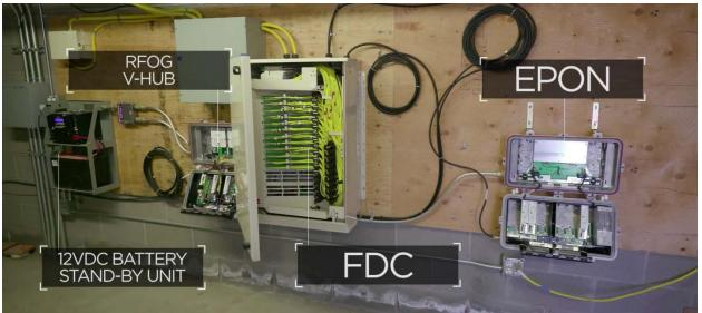
Figure 5 – RFoG / EPON Overlay Actual MDU Deployment
