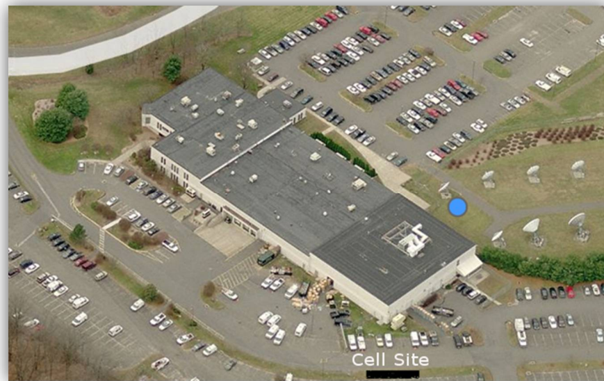
Figure 14 – Berlin, CT, Aerial photo. The black rectangle indicates the Fuel Cell Location.
