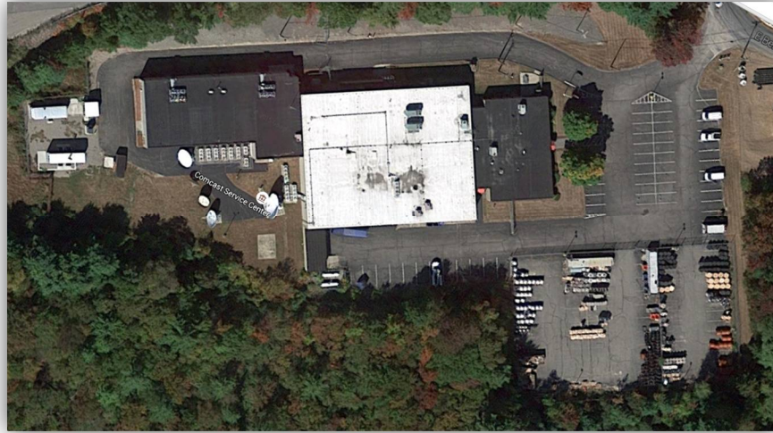
Figure 7 – Foxboro MA, Aerial photo showing white roof material.
