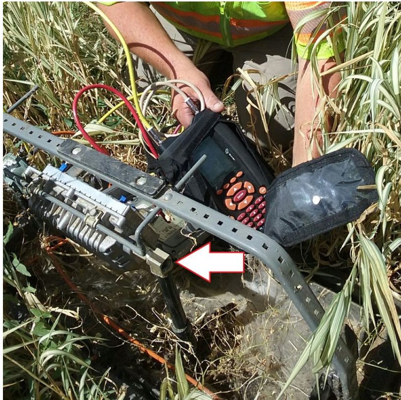
Figure 16 - Location of loose seizure screw at input of amplifier-screw in right angle connector was one-half turn loose
