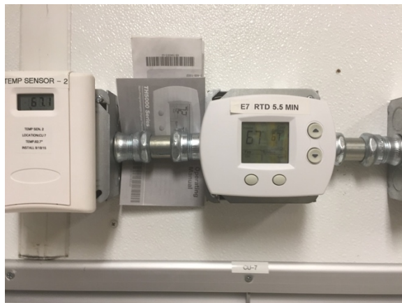
Figure 14 - Site B Programmable Thermostat
